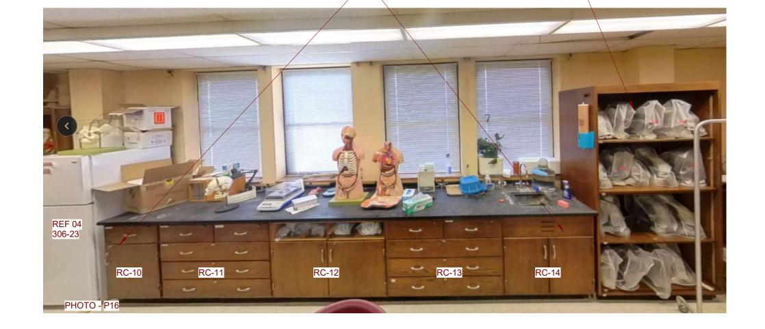
EXISTING WOOD BASE CABINETS TO BE SALVAGED AND RE-INSTALLED IN THE SAME LOCATION. NEW EPOXY RESIN TOP AND BACKSPLASH. —
